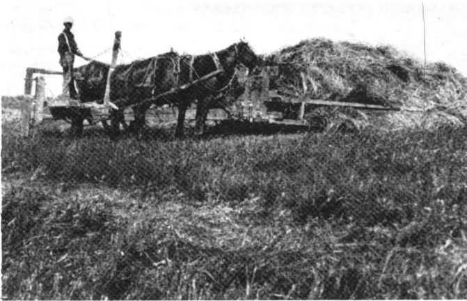
Four-horse buckrake typical of those used to put up wild hay in the Great Basin.
