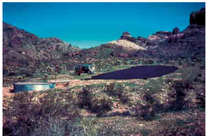
Water-harvesting facility for wildlife drinking water in western Arizona. Photo courtesy of Gary Frasier.
