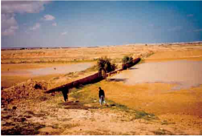
Photo 6. Stone dyke with a spillway across the entire wadi.
