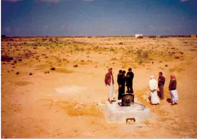
Photo 7. Top of a cistern for storing water from the water-collection area in background.
