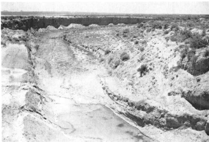
BIA Photo Polacca Wash - 1945. The channel downstream from the newly constructed earth dam built across Polacca Wash to control erosion. Summer thunderstorms not only cut the channel down, but widened it by sidebank cutting. The channel in places is more than 100 feet deep and 400 feet wide.
