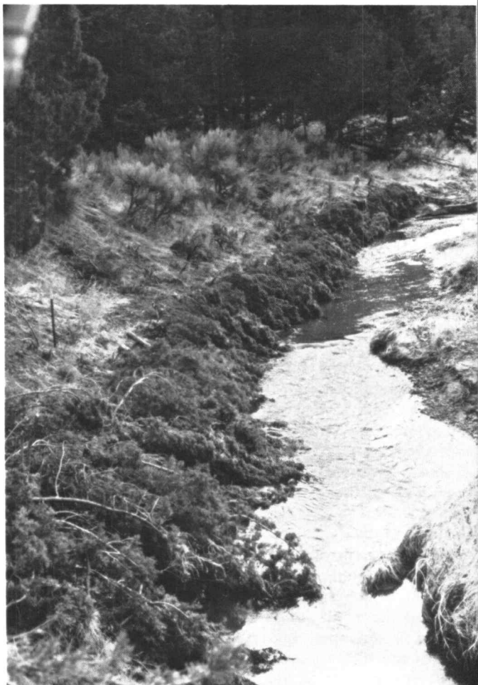
Vegetative riprap made by suspending and securing cut juniper against an eroding streambank.
