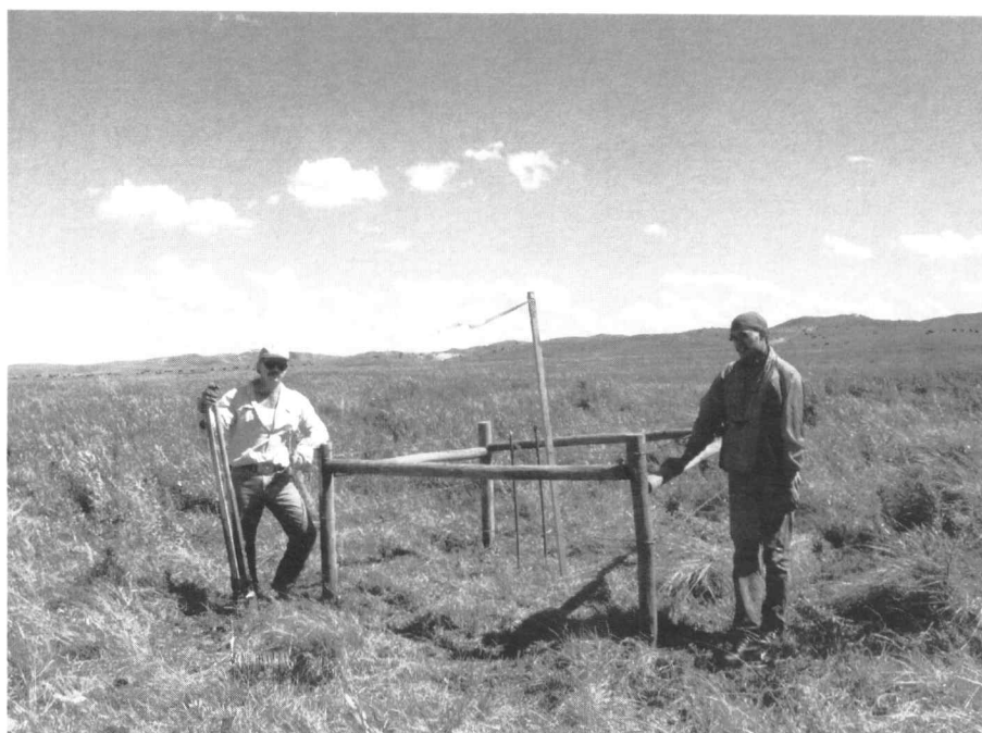
Erecting a protective structure around a pizeometer.
