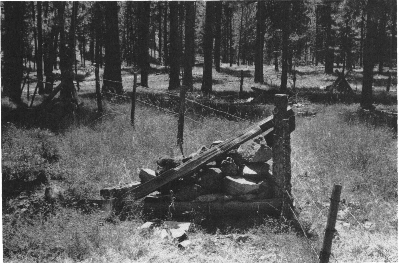
Rock jacks were commonly used in construction of wire fences on the shallow or rocky soils.
