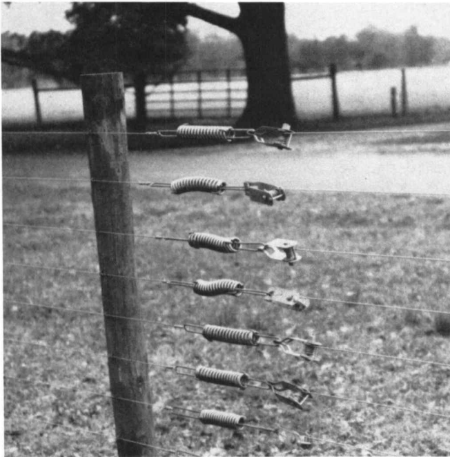
Springs and ratchets used to maintain tension in high-tensile fences.
