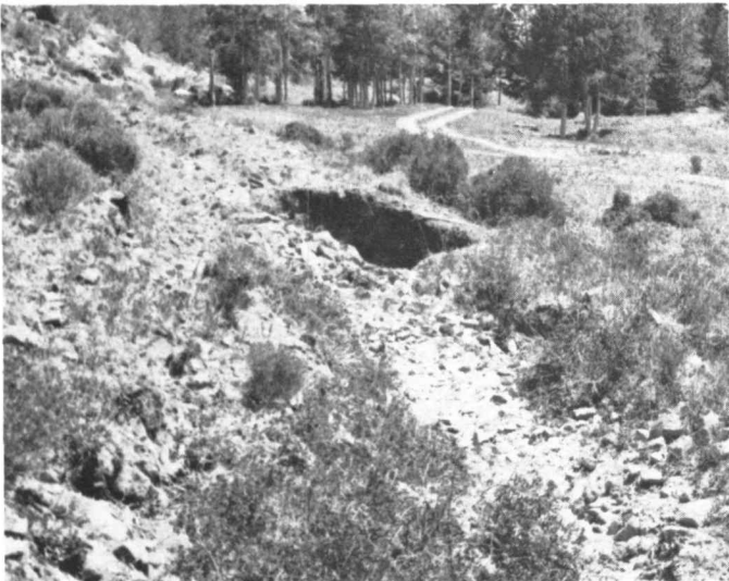
Miles of water transmission ditches dug by hand and horse-drawn equipment collected water on the upper slopes of Thousand Lake Mountain. Most were constructed to supply water to homesteads in the 1800's and early 1900's. Lack of continued maintenance in recent years has led to breaches. Diversion of collected water onto adjacent slopes initiated numerous gullies. One breach and resulting gully is visible in the middle of the photo.
