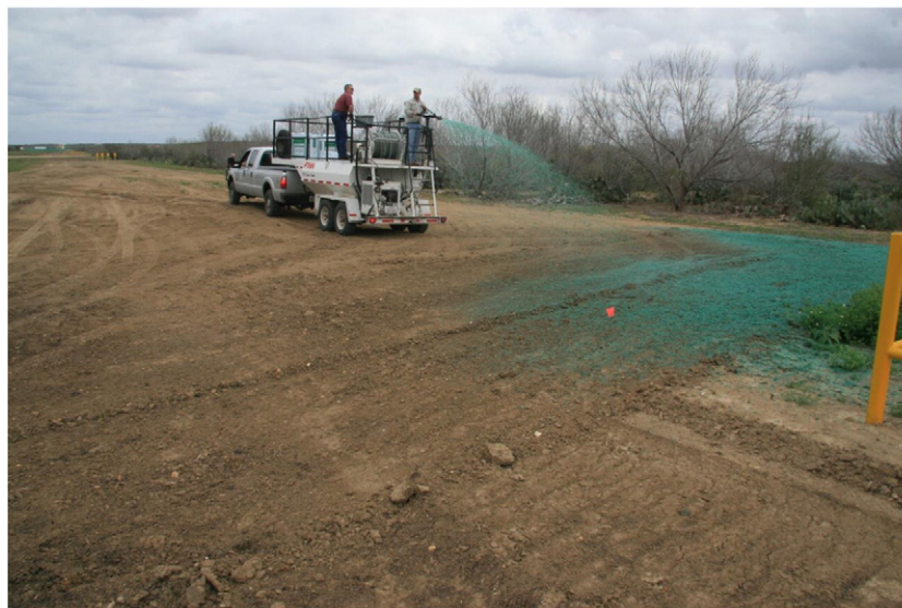
Figure 3. Hydroseeder. Photo by Forrest Smith.
