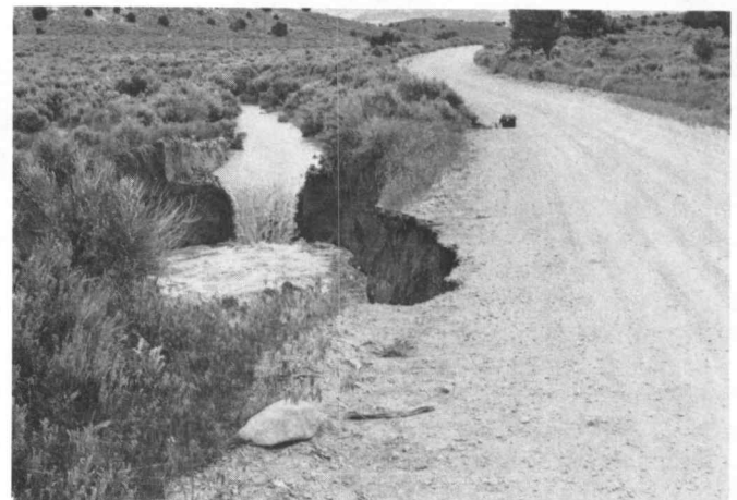
Waterfall at time of last day of observation, June. 15. Fall is now just less than 6 feet. Erosion had taken away part of nearby road.
