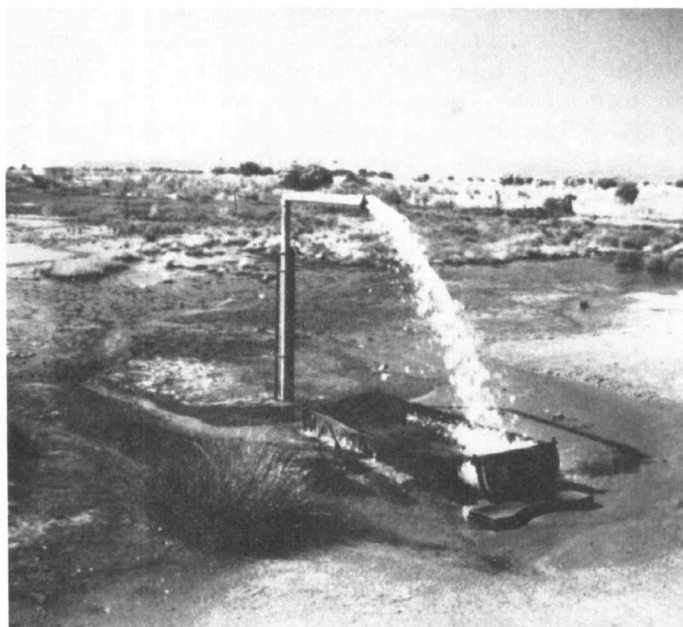
A live bore (artesian well) in northwest New South Wales feeding a narrow ditch which will water livestock for miles.
