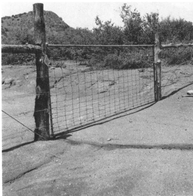
Fig. 9. Used 1-inch galvanized pipe frames covered with hog, chain link, v-mesh, etc. fabric is suitable for predator-proofing gateways. It may be necessary to provide a sill under the gate in friable soil areas to prevent predators from digging under.
