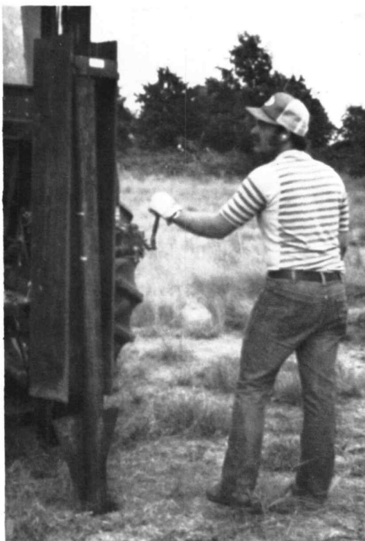
Driving the large anchor plate post.
