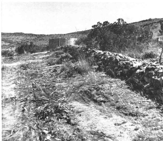
An above-ground gravity flow water system covered with sotal and rock.
