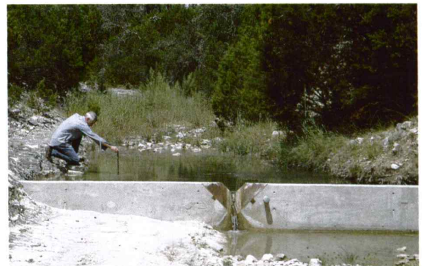
Tom Fillinger, Soil Conservation Technician for the Seco Creek Demonstration Project, monitors spring flow behind a V-notch weir before and after brush management.
