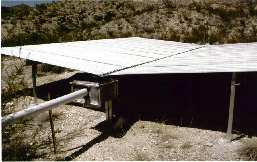
The Black Gap style guzzler with elevated catchment has been successfully used for years. Increased materials and labor make this design somewhat more expensive.
