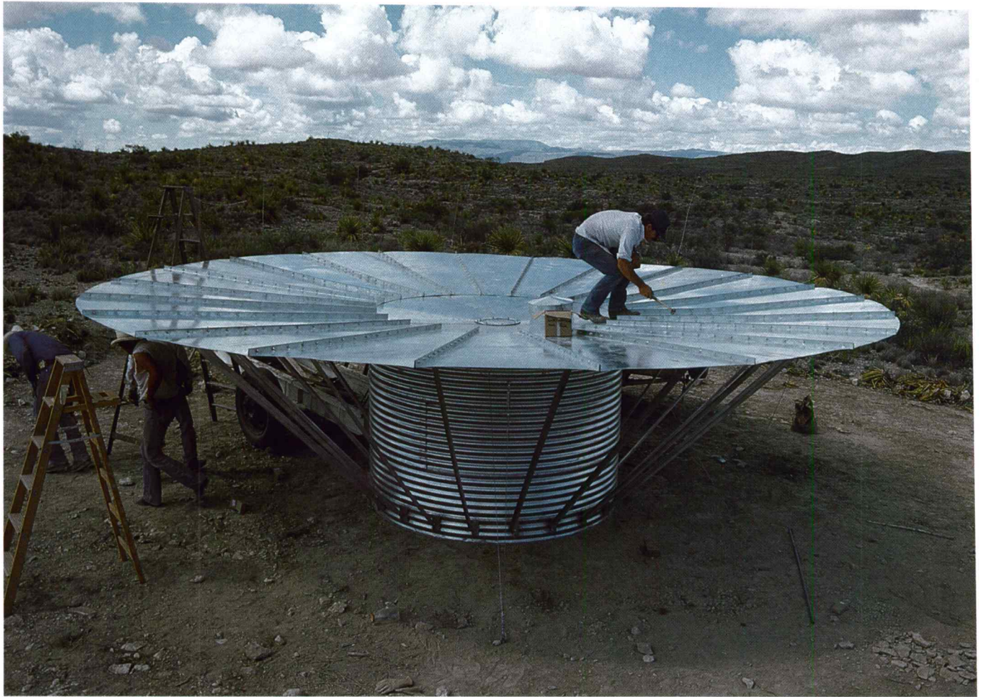
Inverted umbrella guzzler is easily assembled and requires very little site preparation. The 434-square foot catchment requires 8.3 inches of rain to fill the 2,250-gallon tank, making it less efficient than other designs.
