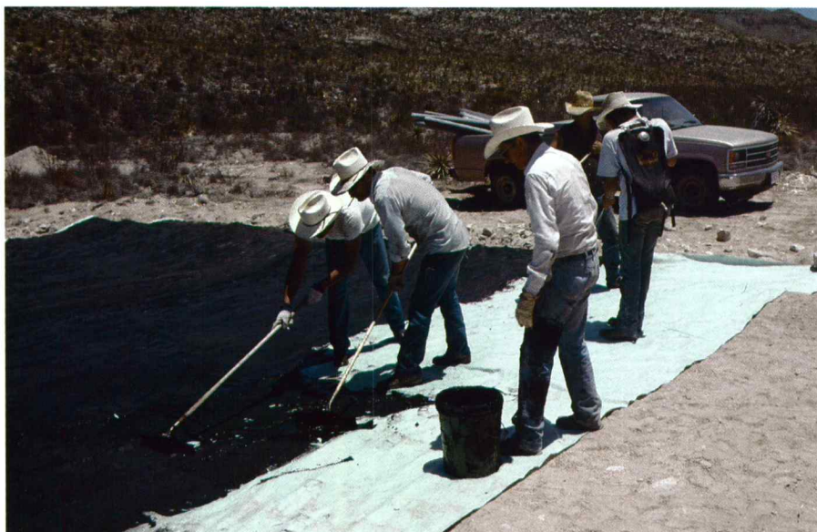
Application of asphalt emulsion to polyester blanket. Blanket must be pre-wetted with water for asphalt to penetrate fabric. Catchment construction required 53 hours of labor.
