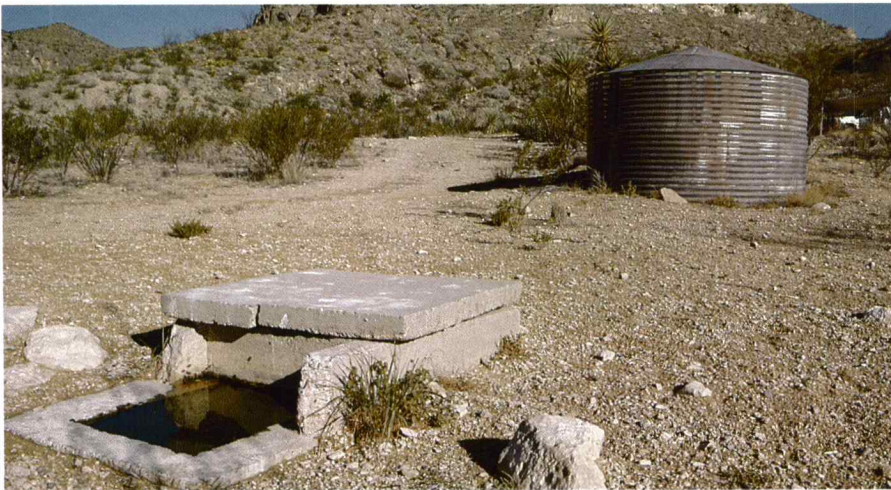
Wildlife drink from a small ground level basin that is regulated by a covered float box. This guzzler has been in use for over 20 years at the Black Gap Wildlife Management Area. Evaporation loss from this drink amounts to only about 100 gallons per year in this 100-inch plus evaporation zone.
