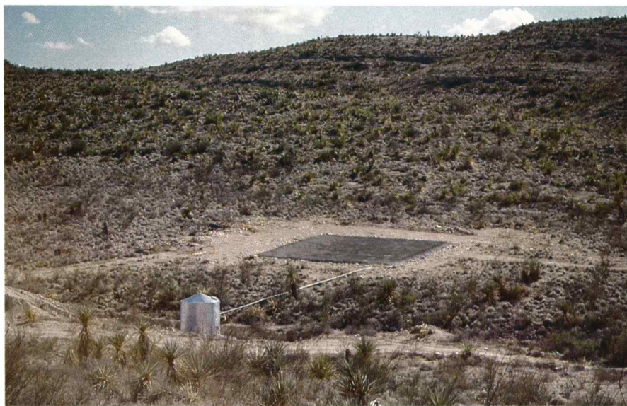
The 1,600-square foot fabric and asphalt catchment will fill the 3,000-gallon tank with 3.3 inches of rain.
