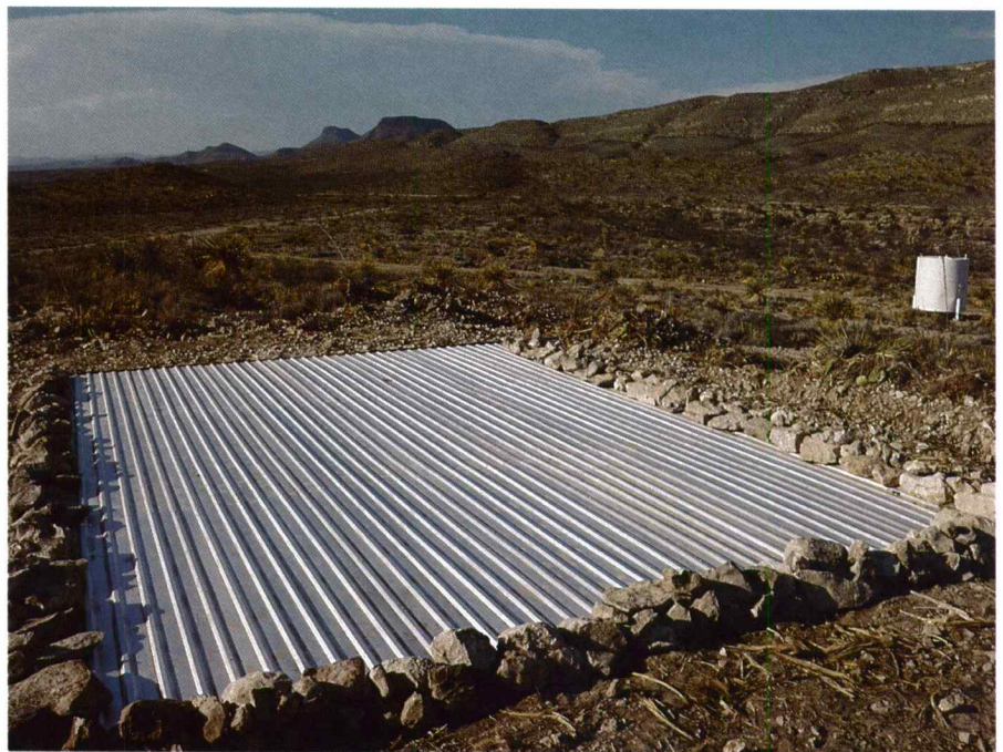
Ground level steel catchment anchored with rock. A gutter and sump divert rainfall to tank using a 4-inch pipe. The 630-square foot catchment will fill the 2,000-gallon tank with 5.1 inches of rain.
