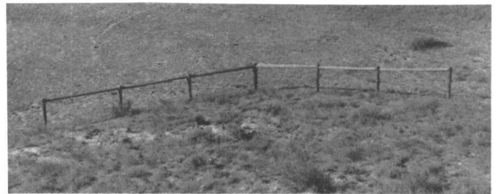
Fig. 9. Using a six-panel brace assembly to increase the resultant effective length of a brace beyond the critical length at a dog leg. impending fence post pullout problem at a dog leg.
