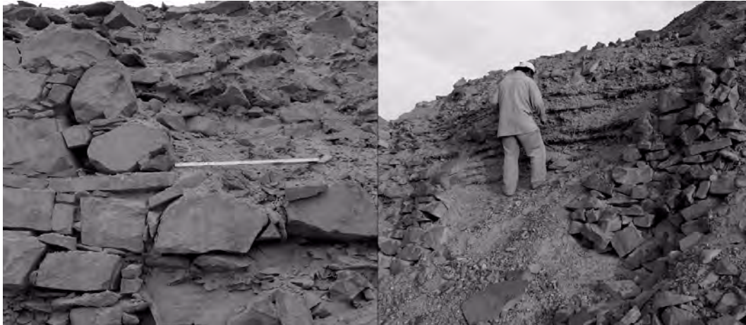
Figure 2 Two dated wall styles from the Fortress of Acaray, showing part of the outer façade and the construction fill exposed by wall collapse: EH style (left) with rock and mortar, and LIP style (right) with plant layers visible. Scale on left is 50 cm. Photos by Brown Vega.
