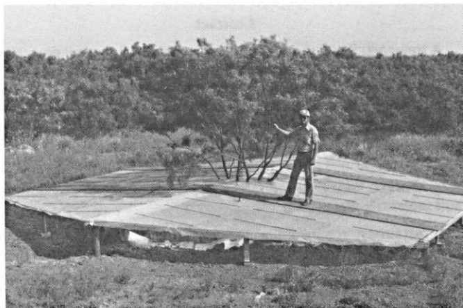
Fig. 4. A completed shelter in place beneath the canopy of a honey mesquite tree on the W.T. Waggoner Estate near Vernon, Texas.
