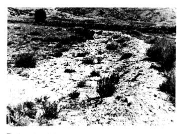
Fig. 1. Roadways had all been made by a grader or bulldozer passing over the site to clear off brush and smooth off surface irregularities. Plant debris and surface soils were windrowed into a berm at roadedge. There had been no attempt to form gutters or elevate roadbeds. Plant life persisted in the center of all roads sampled.
