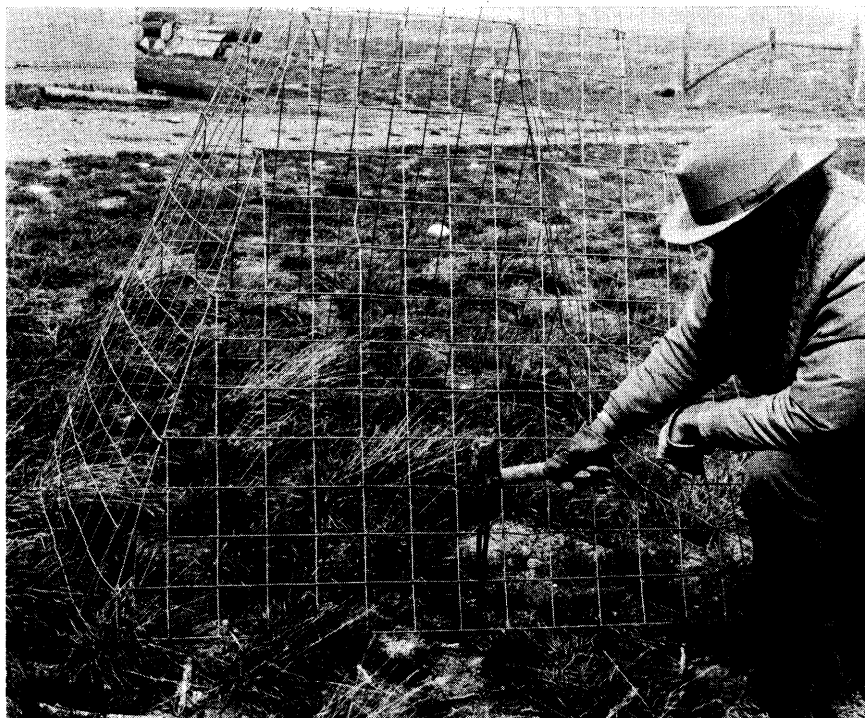
FIG. 1. Installing pyramidal cage of 4- by 4-inch mesh galvanized 10-gage wire.
