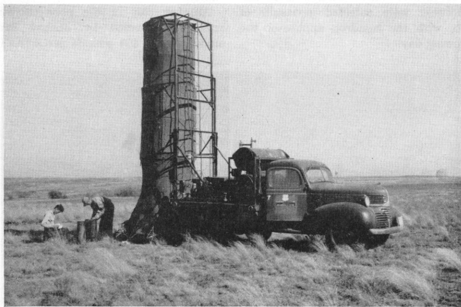
FIGURE 1. Raindrop applicator in operation on range land.
