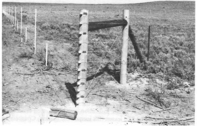
Fig. 7. Detail of corner post.
