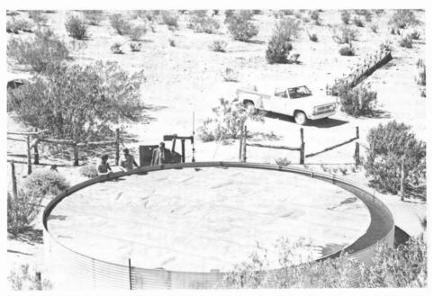
Fig. 3. Thirty-foot diameter floating cover on water-storage tank near St. George, Utah. The cover should be fabricated to fit the tank more closely than this one does.
