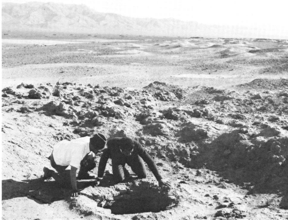
Fig. 3. Opening of ventilation and access shaft of a qanat at Estahard. Other shafts are indicated by spoil piles in the background.
