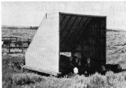
FIG. 2. Steers using north-facing shade. Note steep pitch of roof to permit radiant heat from the animals to be absorbed by the cool, "black," north sky.
