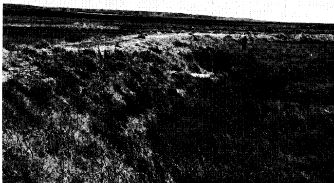
FIG. 4. Ponding has been eliminated in the Coal Creek Spreader near Terry, Montana by draining water through culverts in the dikes (left). Earth for the carryall-built dikes was borrowed outside the flooded area except at sites (right) where water storage for livestock was desired.
