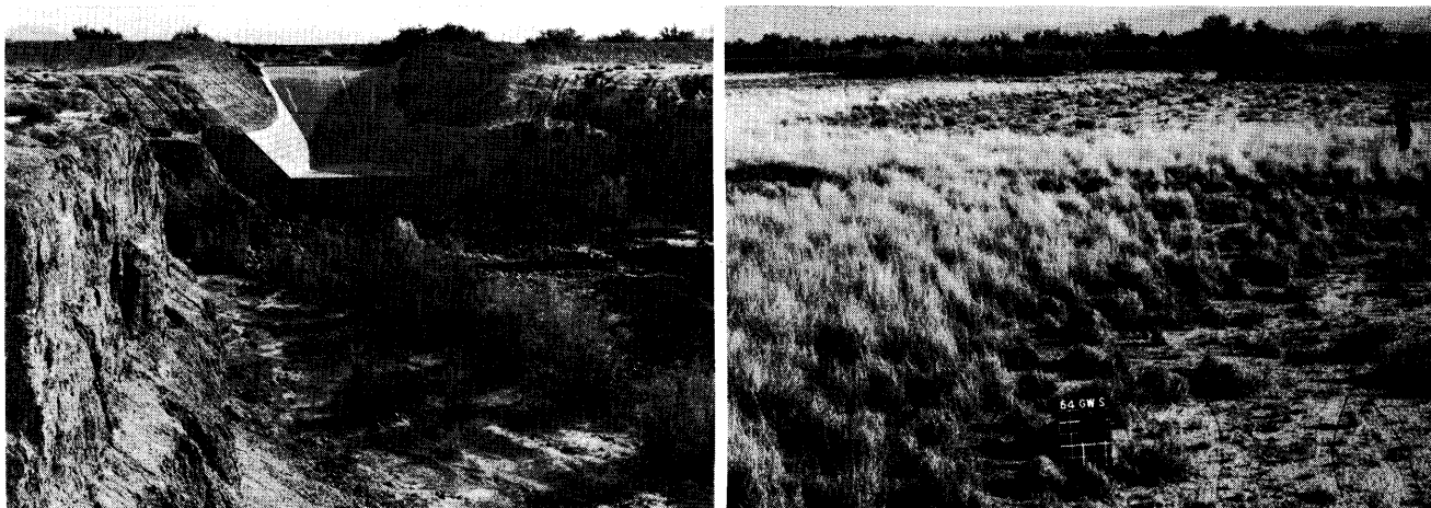
FIG. 5. The concrete drop structure (left) protects the large earth dike across Goat-Well Wash, south of Solomon, Arizona; while water is drained through the dike in culverts at a distance from the gully (right) to prevent re-entry into the gully.
