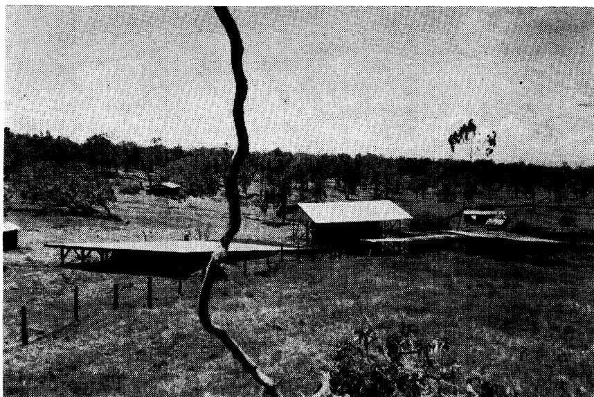
FIGURE 6. The catchment tanks at Pauahi under galvanized steel roofs, which gather the water during the rainy season and carry it to the tanks which are covered by the roofs. (Photo Soil Conservation Service, USDA)
