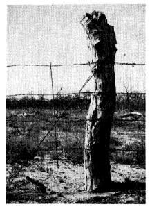
Support posts are placed every 1/4 mile. The support consists of a deadman anchor set 2 feet in the ground and attached to the post with No. 9 smooth wire. The twisted wire stays, as shown, are placed every 10 feet to keep the animals from forcing the wires apart.
