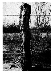
Line post in the suspension fence. The  $12\frac{1}{2}$  gauge wire is fastened to the post with a  $\frac{3}{16}$ -inch galvanized plate, 1 inch long, held in place with two eight-penny nails driven through holes punched in the plate. Staples are not satisfactory for holding the wire to the line posts in this type of fence.
