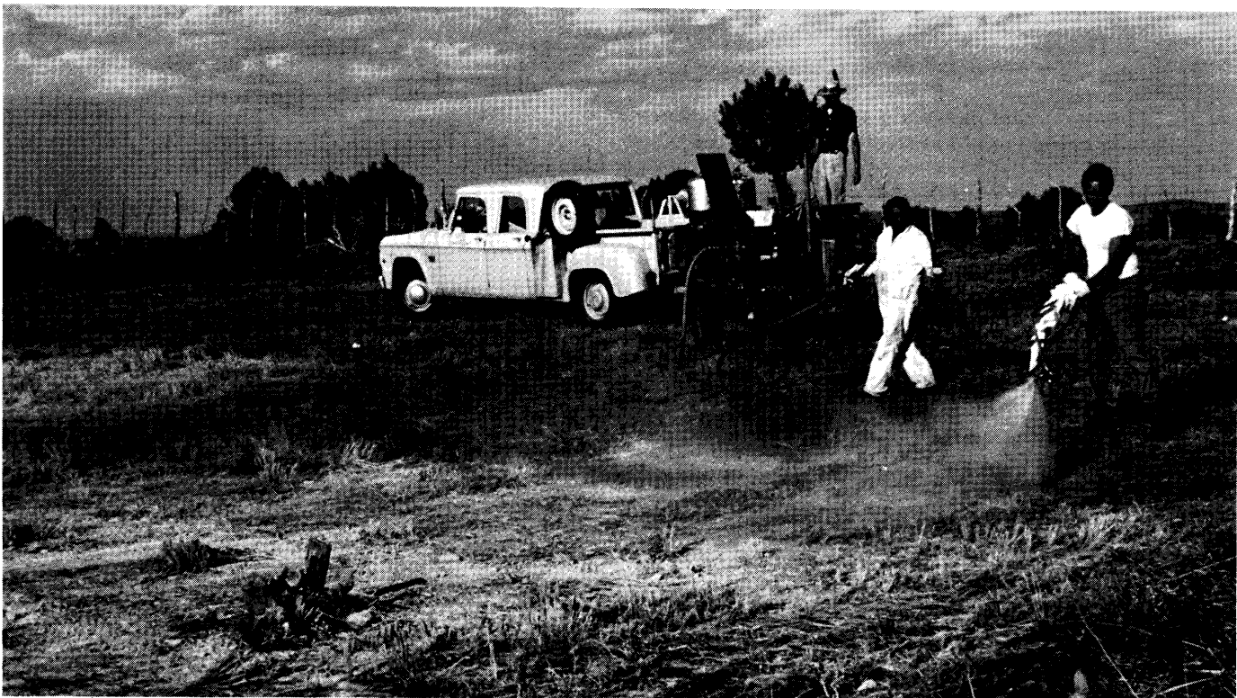
Fig. 3. Application of paraffin wax to a catchment on the San Carlos Indian Reservation in Arizona.
