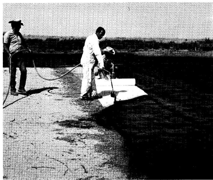
Fig. 4. Installation of an asphalt-fiberglass water harvesting catchment.
