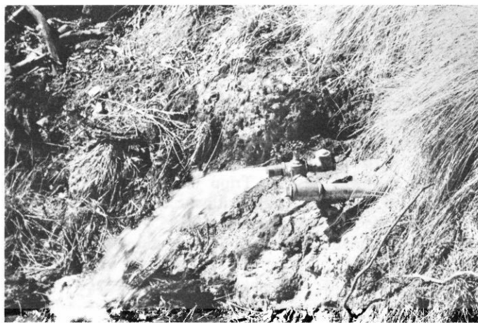
Fig. 1. A completed horizontal well on the San Carlos Apache Reservation test yields over 50 gpm.
