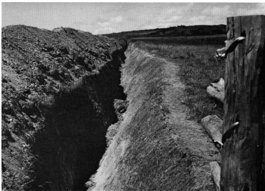
FIG. 3. Game-proof ditch and fence under construction, showing the dirt piled on the ranch side. A four-foot fence will be erected on the dirt and the ditch covered with cut bush.
