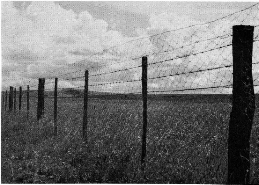
Fig. 4. Five-foot high wire netting fence to keep hyena and jackal out of a 23,000 acre area.
