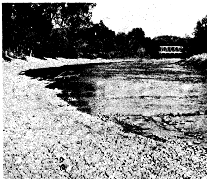
FIG. 1. Bulldozed gravel bed for salmon spawning on Battle Creek, Gover Ranch, Shasta County, California.
