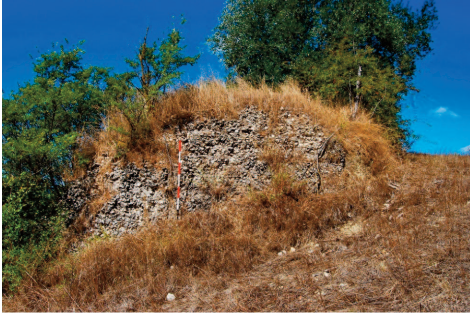
FIGURE 3: Lugnano in Teverina (Italy), cistern of Poggio Murlo, eastern side.
