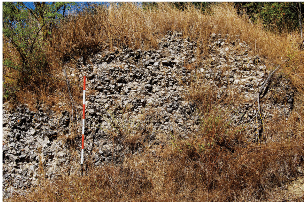
FIGURE 4: Lugnano in Teverina (Italy), cistern of Poggio Murlo, front view of eastern side.
