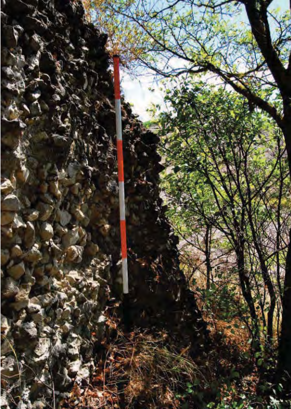
FIGURE 5: Lugnano in Teverina (Italy), cistern of Poggio Murlo, southern exterior facing.
