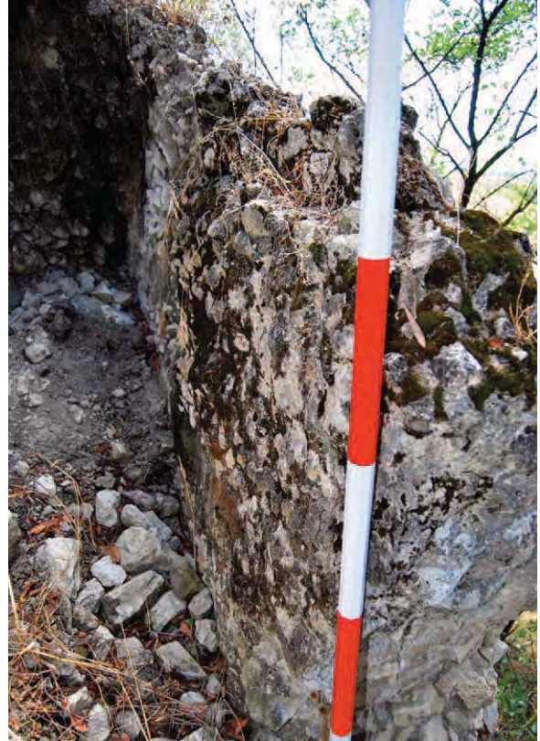
FIGURE 6: Lugnano in Teverina (Italy), cistern of Poggio Murlo, southern interior wall.
