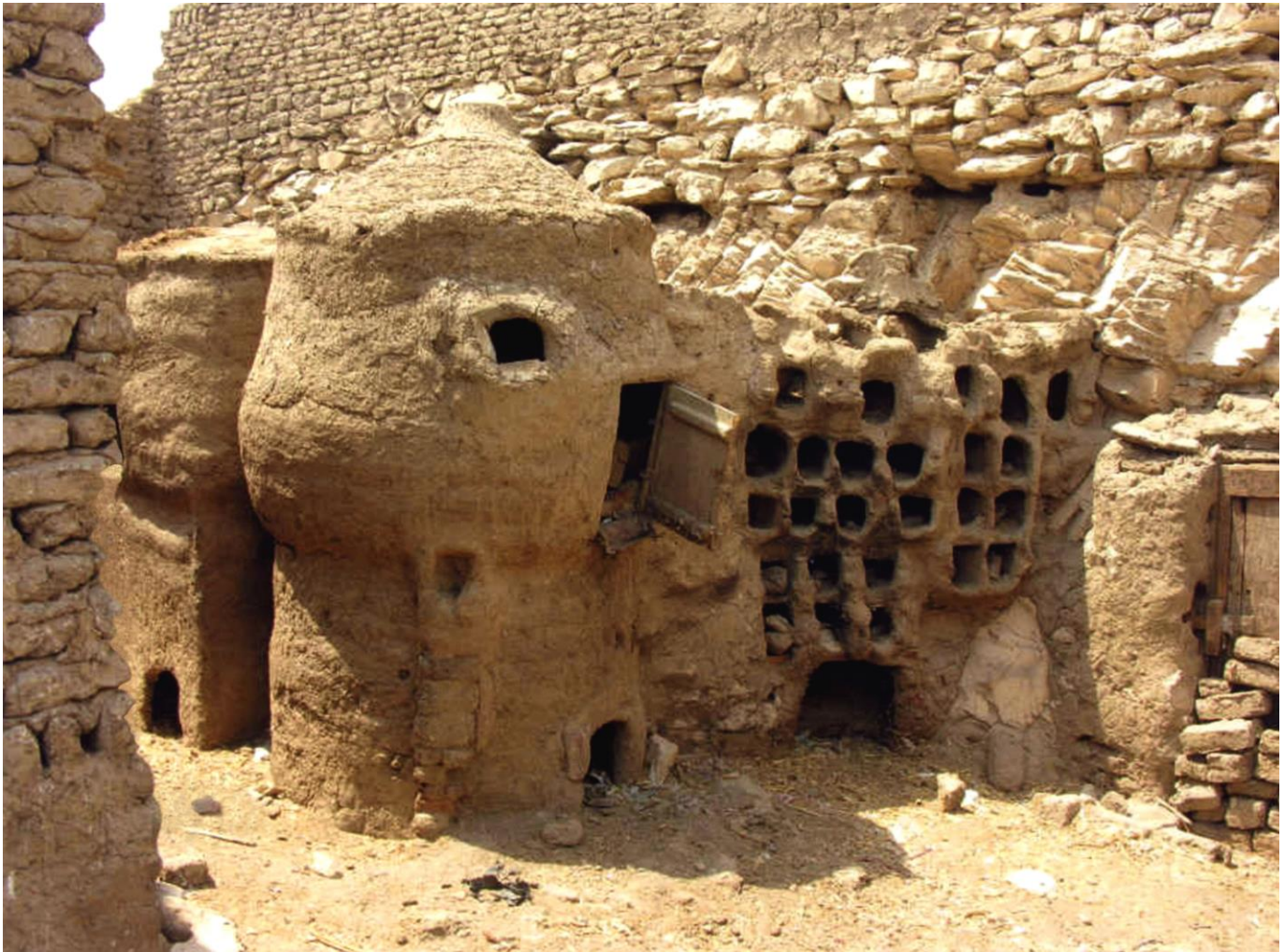
Figure 10: A variety of grain cylinders and domestic storage spaces shaped from mud complemented al-Qurna’s vernacular architectural assemblage of tomb, tomb-forecourt, and house. Elements of all of these are visible in this image of one spectacular example that demonstrates the beauty and versatility of mud architecture. Much of this vernacular storage had already fallen into disuse as a result of changes in agricultural production (from wheat to sugarcane cultivation) and the uptake of modern consumer goods. Nevertheless, there will be those that remain in tomb chambers that once formed part of contemporary Qurnawi dwelling spaces. Photograph courtesy of Caroline Simpson and Elina Paulin-Grothe.
