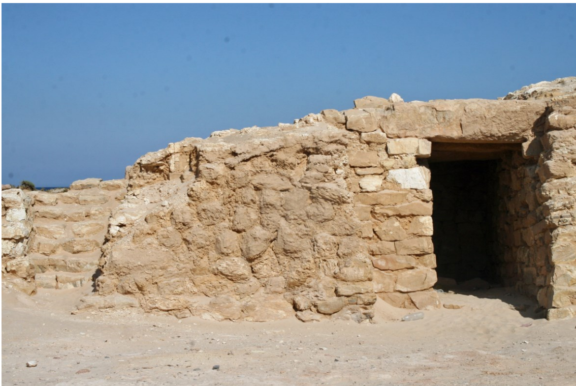
Figure 18: 2008 view of the fort's western interior with the stairway, retaining wall, and the unblocked/open eastern end of the entry passage (Photograph: P. Carstens)
