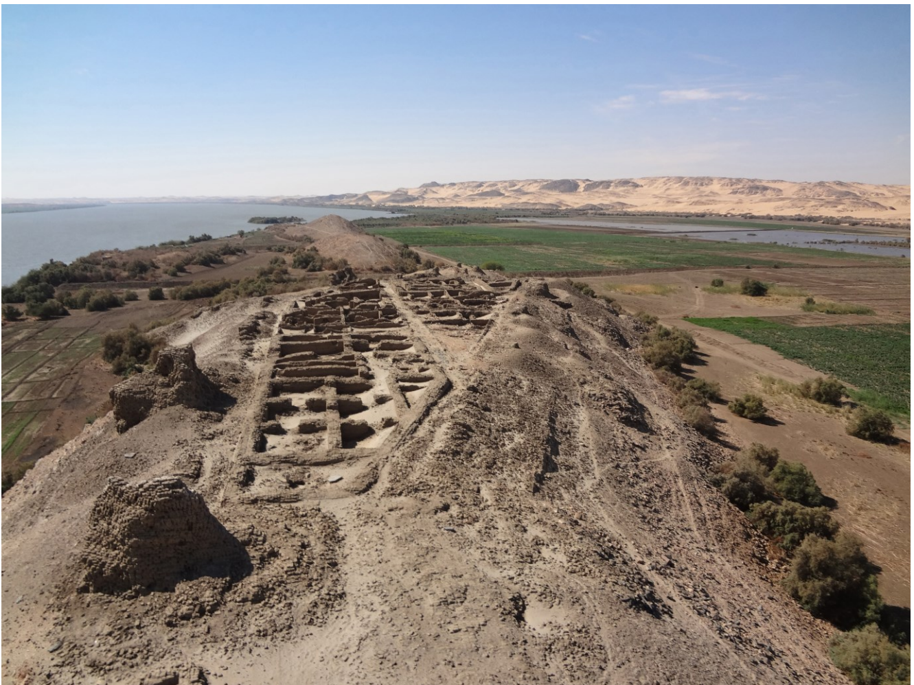
Figure 1: The island of Uronarti looking approximately south. In the foreground is the fortress itself, with the granaries in the near section. (Kite aerial photograph, authors)
