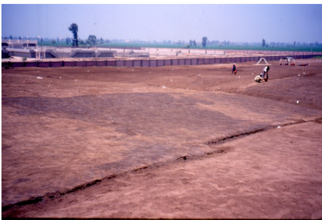
Figure 15: Looking northwest at the East side of the buttressed outer enclosure wall and water filtration plant in the background. Photograph by G. Mumford.
