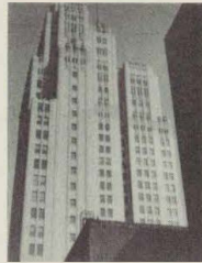
Telephone Building, San Francisco, 1928 81:111:098
