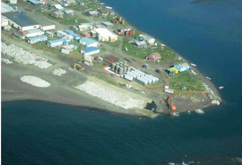
Figure 2: Rock revetment project under construction, Kivalina 2008. Source: author
